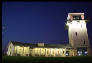
Falls Park Tower & Visitor's Ctr
